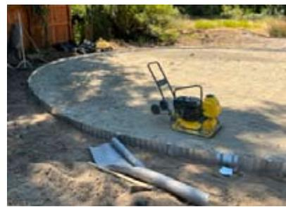
Gravel arrives on July 26. Perimeter ring is set, gravel is spread and compacted
